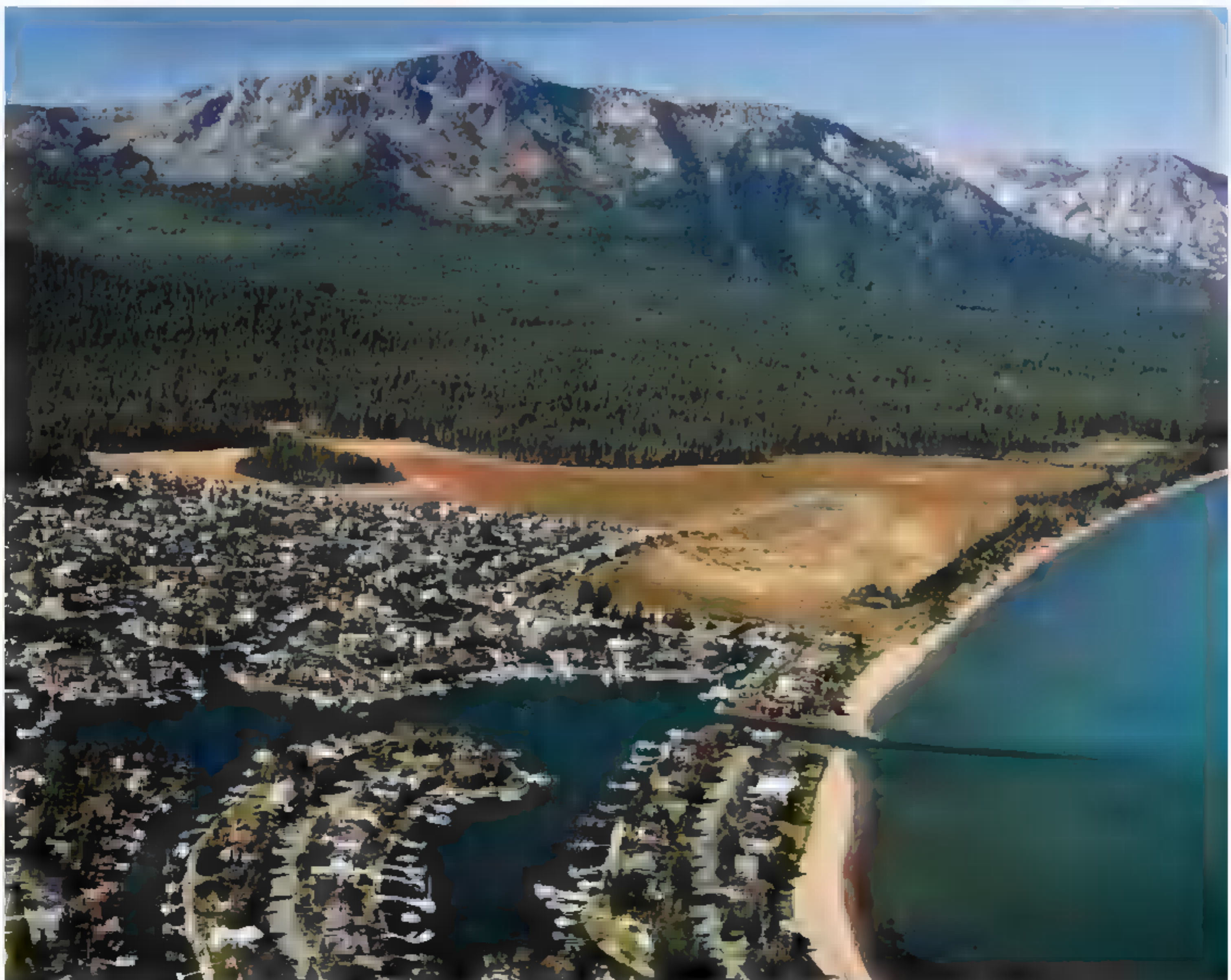
Runoff from developments is blamed for dimming Lake Tahoe's brilliant blue water.
